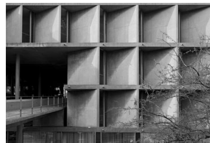
Fig. 9: Brise-soleil in Le Corbusier's Mill owner's Association Building
